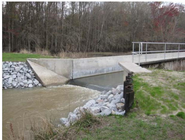
Flume in Canal
