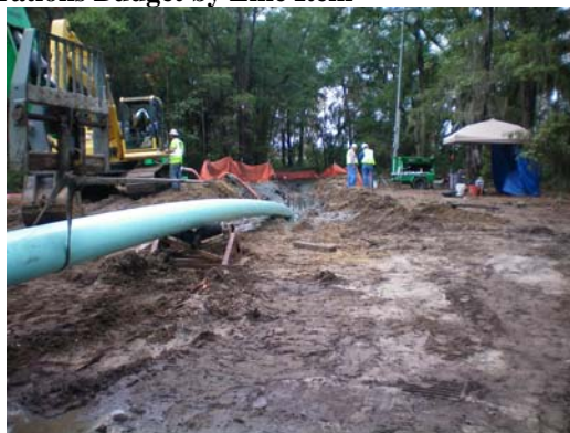
Fusible PVC pipe near the Archers Creek Site
